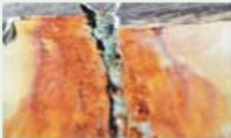
STAINLESS STEEL PIPELINE
